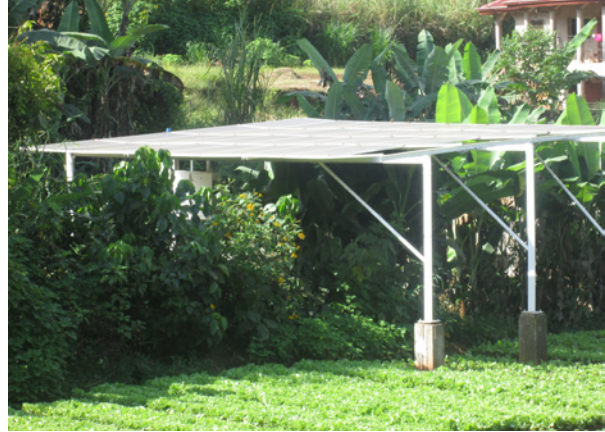
Picture 19. PB funded solar panel installation for drinking water pumping and distribution, Nyom neighbourhood © Yaoundé Commune 1
