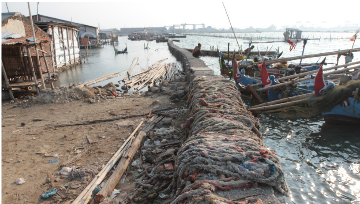
Picture 4. Flood retaining embankments built by local government to withstand flooding. However, the tidal flood keeps affecting community's settlement. Semarang, Indonesia, Tambor Lorok community © Kota Kita
